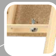
A metal latch keeps the hatch in the closed position.
